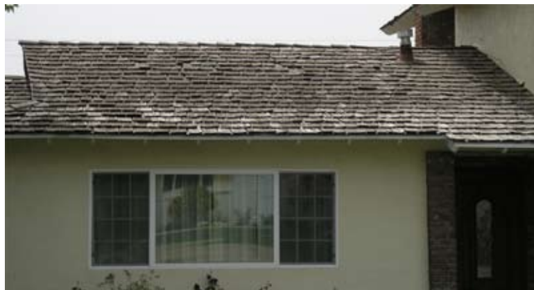
Figure 1—Cedar shake roof.
