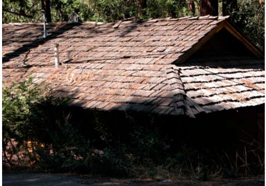
Figure 2—Cedar shake roof.
