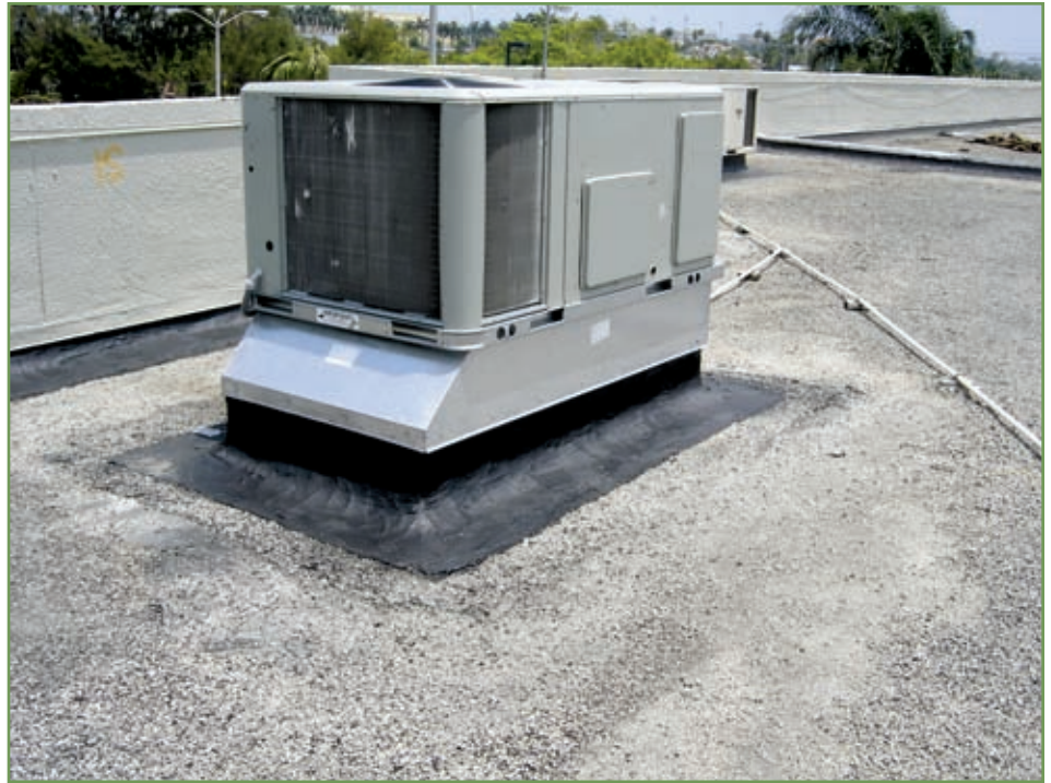
Metal counterflashing over base flashing repair.
