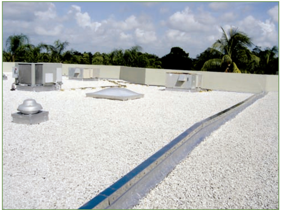
Fully restored roof-pitch pan, power vent, HVAC, skylight, and roof divider.
