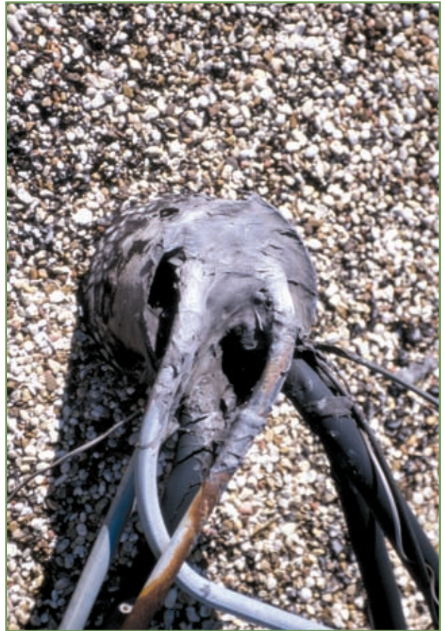
Challenging multiple pipe pitch-pan detail.
